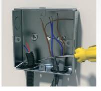
Depending on the type of mat supplied, the cold tail (black lead) may have either a solid earth cable or an earth braid wrapped around the internal cores, this needs to be unbraided by using a screwdriver and pulling down the braid to separate the strands. These can then be twisted into a single strand.
